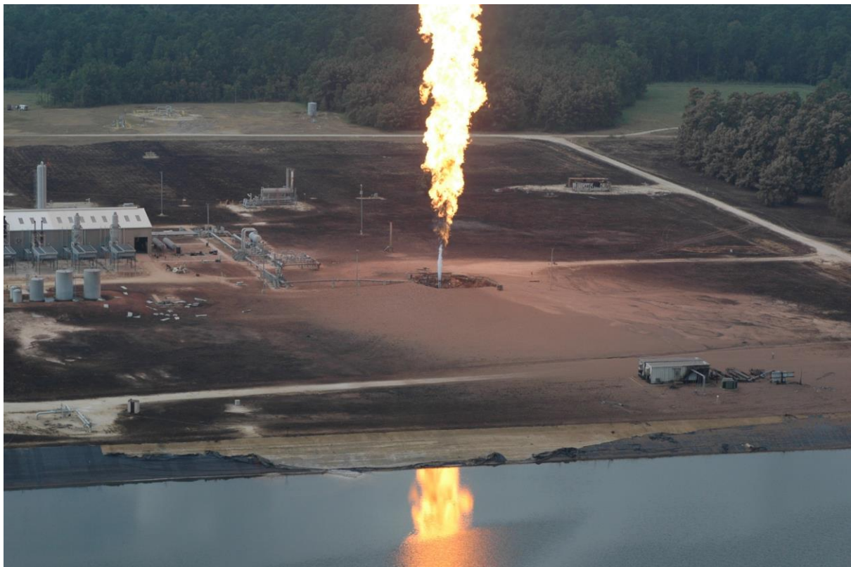
Figure 41. Blowout and fire at Moss Bluff.
