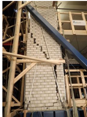
Figure A.10 Damage at the end of the test performed at TU Delft on a full-scale assemblage representing the load-bearing structure of a terraced house. From [Esposito et al. 2018].
